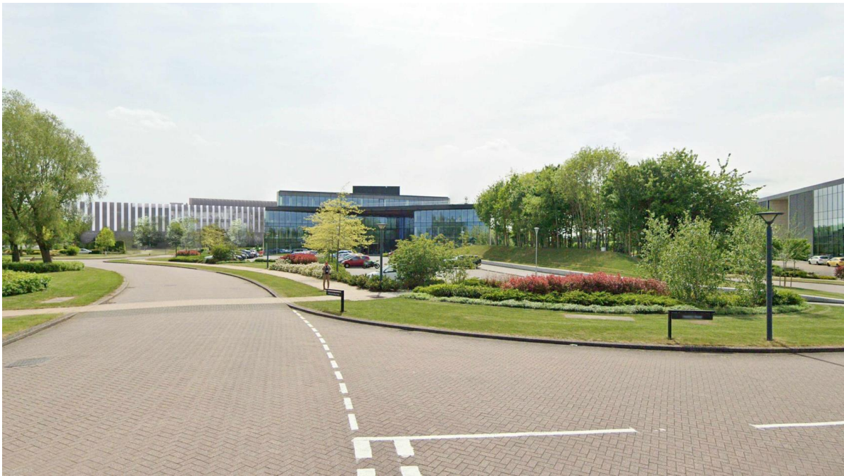
Figure 3: View of building 3 from Heatley Road
